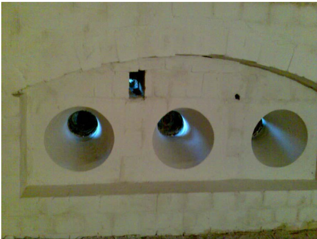
Burner blocks after coating with ESPON
