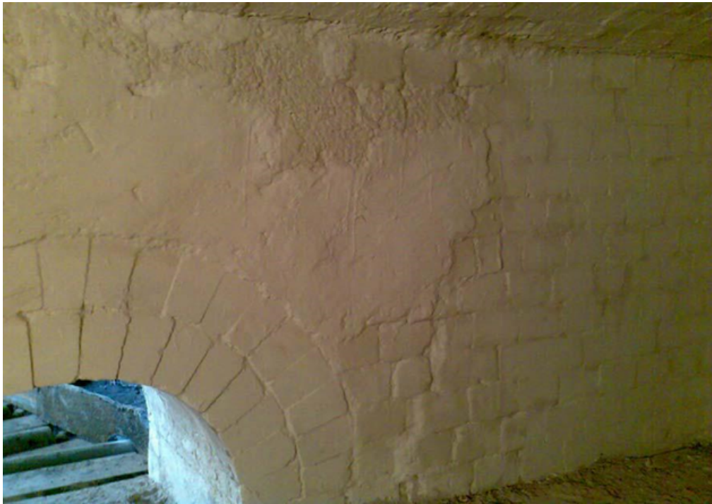
Refractory lining after coating with ESPON
