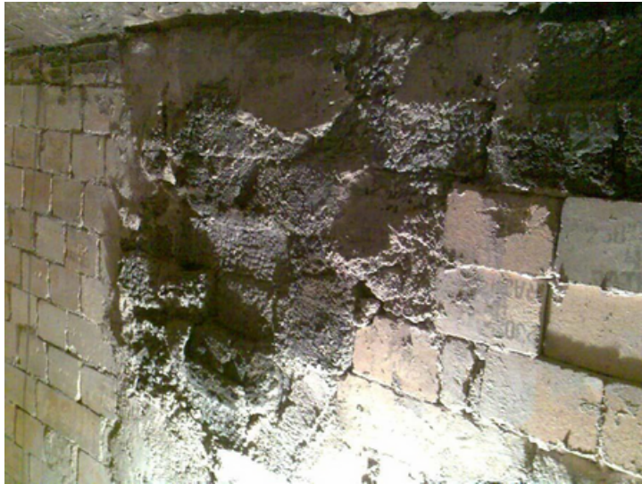
Refractory lining before coating
